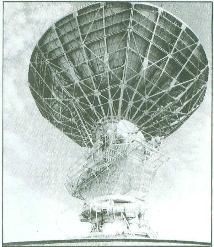
Left: Engineer working on a semi-electronic exchange. Right: Satellite receiving station.
